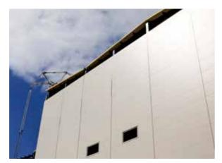
Installation of the façade cladding. The three production halls have external sandwich panel cladding that is 30 m tall.
